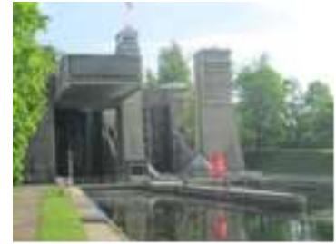
Waiting to exit. Note how high the water line is on the Lock wall.
