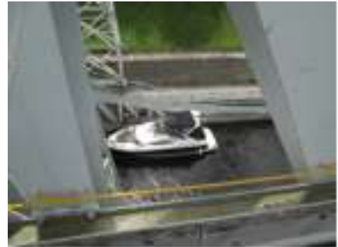
Looking down from the Kirkfield Lift Lock
