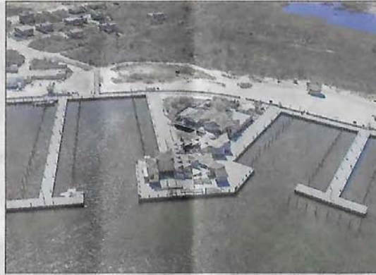
The Watch Hill marina is to reopen Friday. Damage to the substructure added to the cost and time of the post-Sandy repairs.
