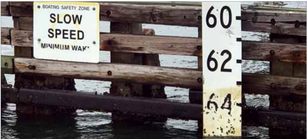
Bridge height board
